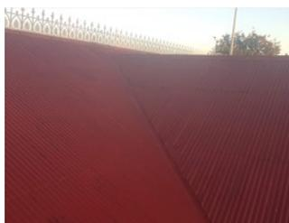
Very fine decorative cast iron filigree ridge capping. The corrugated galvanized roof sheeting has been painted to extend longevity of the product. The ridge capping and sheetings are rusted at the edges, lifting, and allowing water to enter below into the seating area, as well as between sheets.
