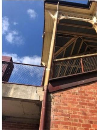
**View of the rear walls mortar joints are loose and eroded.**
