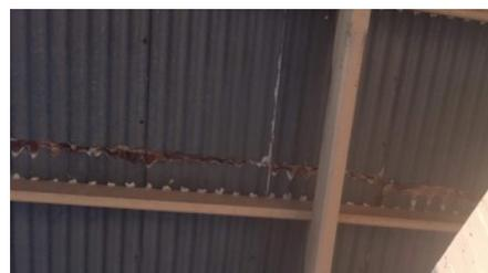
Repairs to corrugated iron roofing should be with galvanized corrugated iron to the original profile and thickness and using fixings to match the original. If possible, sheets in good condition should be retained and new rolled corrugated sheets to match existing profile, thickness and lengths. There are local manufacturers, use of 9mm thick galvanized sheeting.
