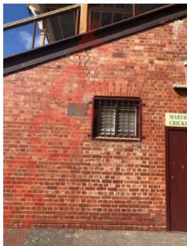
View of the northeast - corner where the timber post is leaning to the west. There is a visible lean to the west of the north-east corner post. This is the site of previous alterations and settlement. The cause is unknown. Future maintenance is associated with repair of the masonry wall described below.
