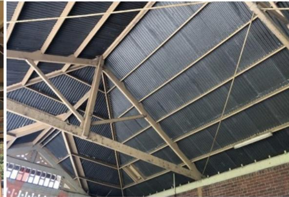
Structural timber, series of roof trusses support the main hip and five gables.
