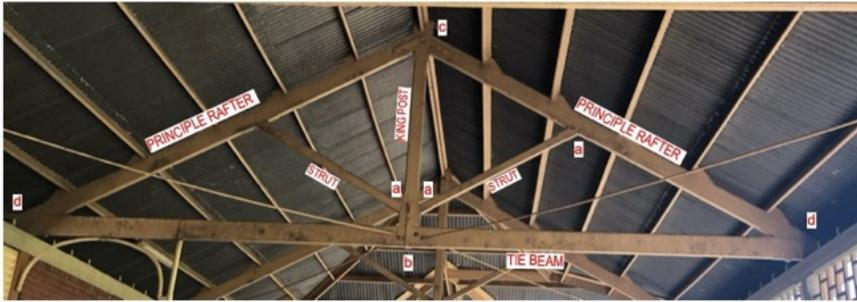
NOTE: FRAMING SIZES HAVE BEEN TAKEN FROM LASER SCAN BUT SHOULD BE VERIFIED ON-SITE
