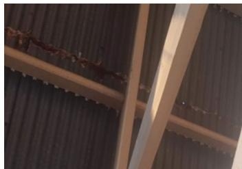
View showing damage and deterioration to the galvanized roof sheeting particularly at the overlapping areas. Due in part to coating failure and corrosion of the metal, including entrapment of moisture between the layers of sheets. This in turn will reduce the structural strength of the sheets.
