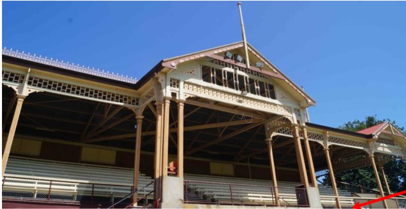
It is recommended that all missing decorative timber detailing is reinstated. Loose timber decorative details have been removed and stored at the Council depot for safe keeping and safety. 1:1 scale dimensioned sketches should be prepared for reconstruction and replacement exactly like for like. This includes replacing the balustrade.
