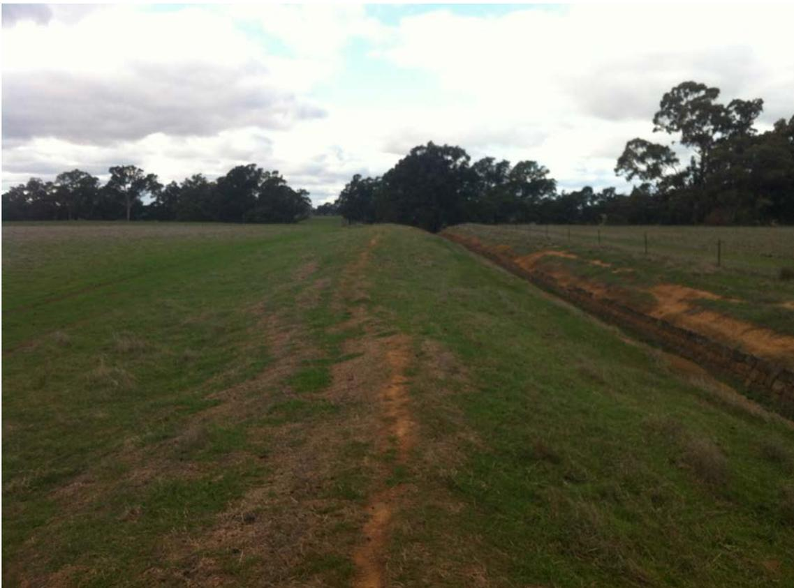
**Figure 7.** Section of the proposed infrastructure corridor within 200 m of McCallum Creek demonstrating the significant ground disturbance caused by drain construction.
