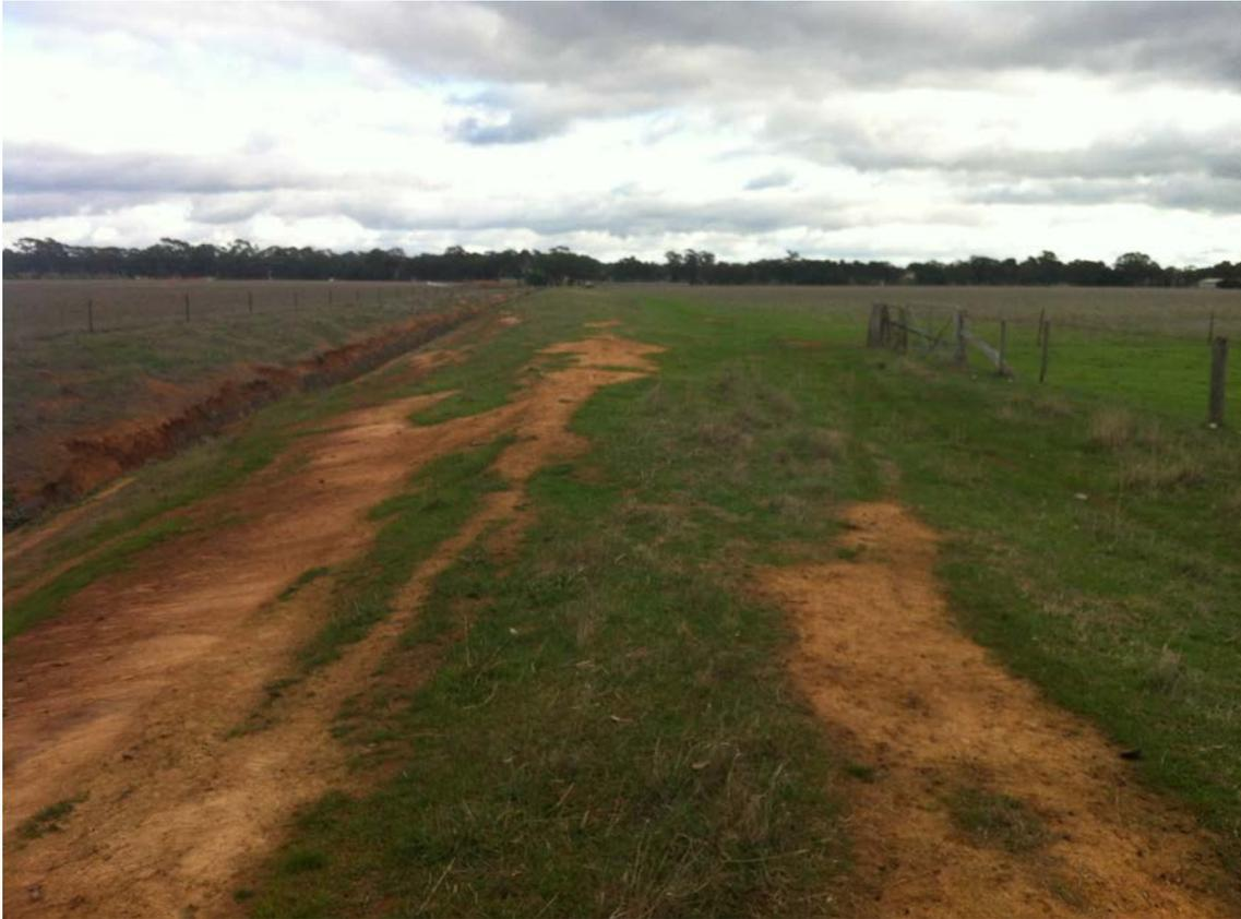
**Figure 6.** Section of the proposed infrastructure corridor within 200 m of McCallum Creek demonstrating the significant ground disturbance caused by drain construction.
