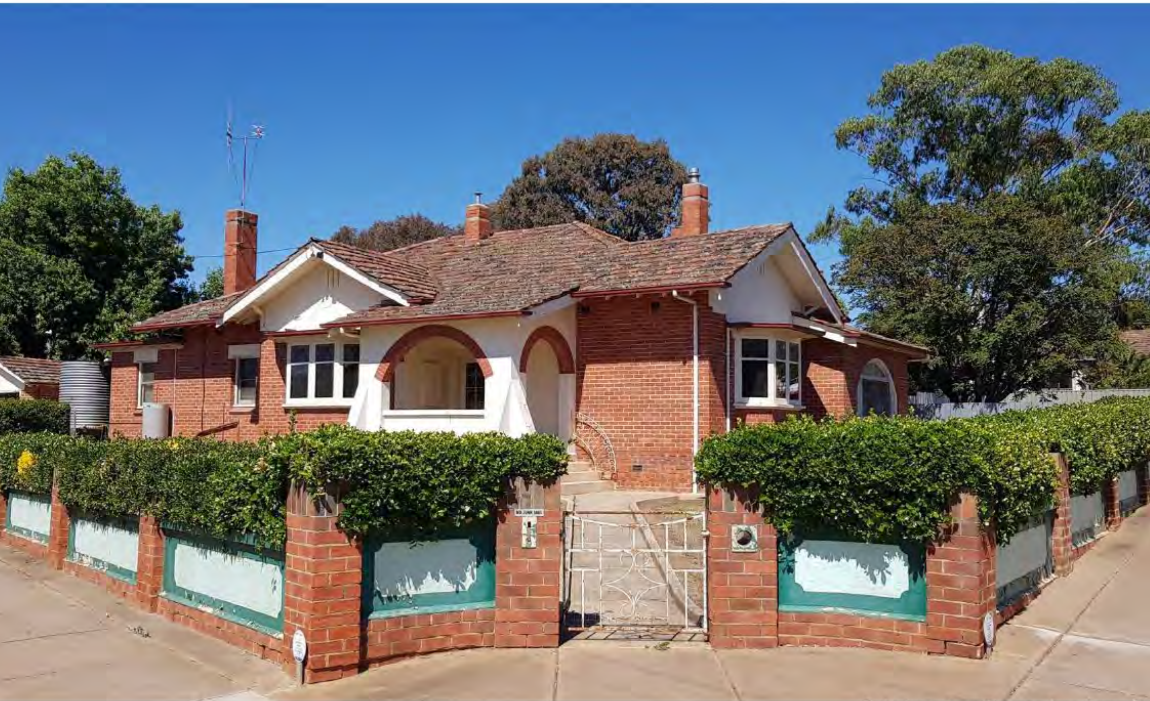
Existing dwelling to be demolis
