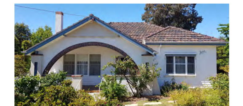
8 NO. 5 NIGHTINGALE STREET - EXISTING WEATHERBOARD HOUSE
